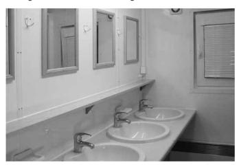
BATHROOM - on the right side there are two shower stands with a sliding door. The area between the two shower stands provides enough room for storing one's outfit, clothes hooks, and a bench. Four washbasins with mixer taps are attached to one board. Each mixer tap is connected to a flow heater. Above the basins there are four mirrors, two 230 V sockets, 5 towel hooks, a shelf for
