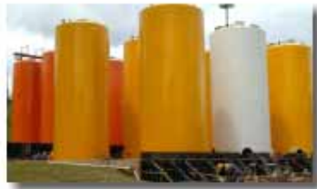
Silos and tanks
