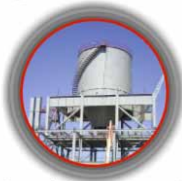
Silo - Savannah Cement Company - USA
