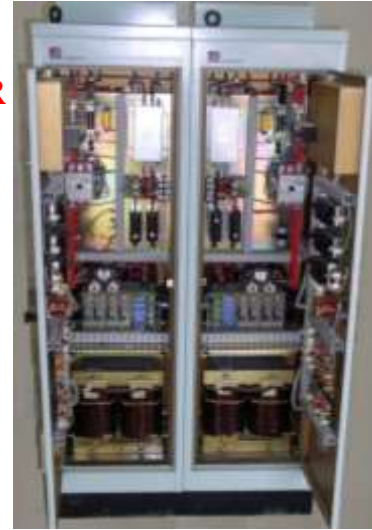
STATIC FREQ CONVERTER
