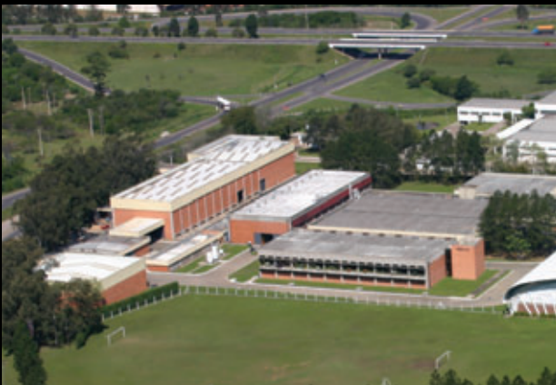
Constantly growing since 1977, the Digicon group has 33 000 sq meters of built manufacturing, engineering and administrative areas.
