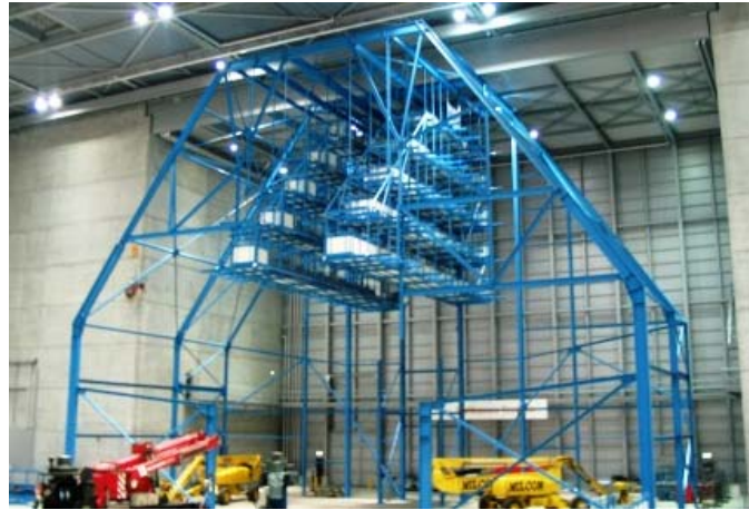
A 380 Taildock with elevator and cranes
